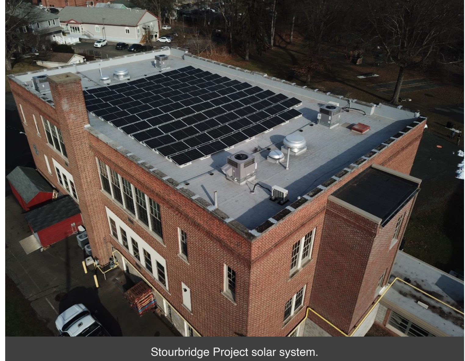
Stourbridge Project solar system.
